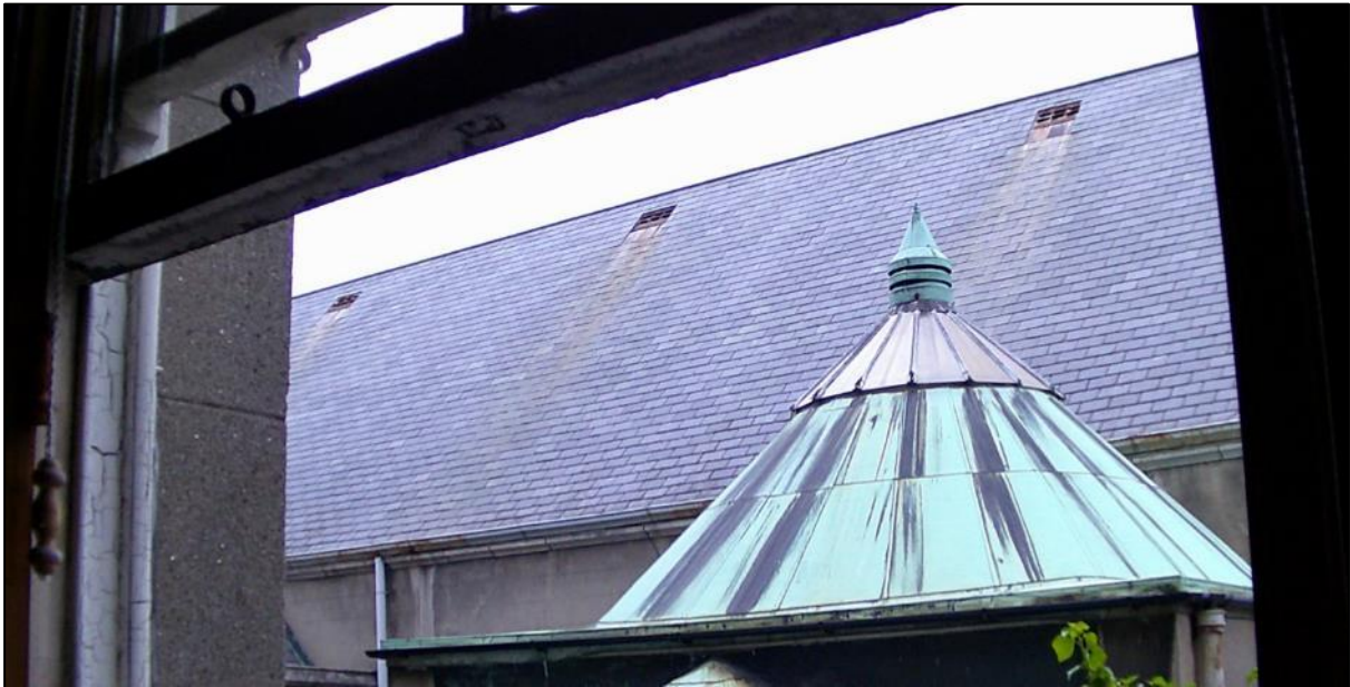
Figure 8.7: View from VP3 facing southern side of the Chapel (Source: DNV).
