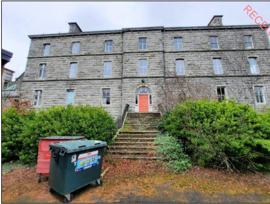
Figure 8.30: Tabor House (Source: DNV).
